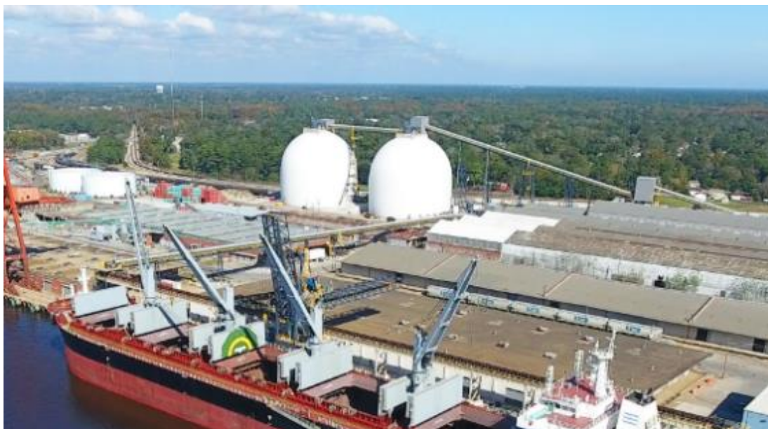
Enviva storage and shipping at the Port of Wilmington
